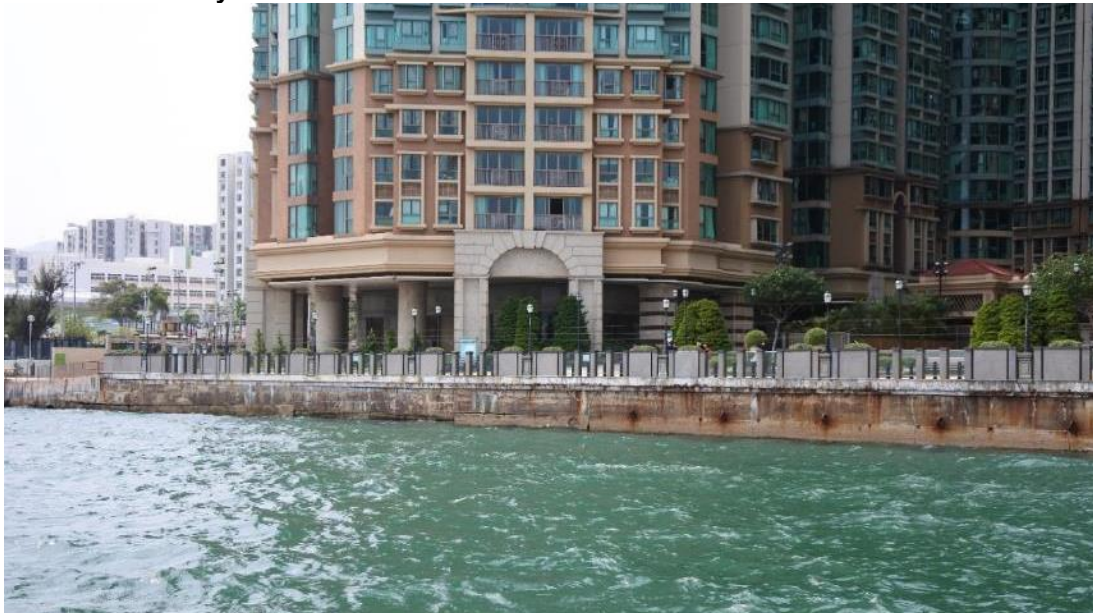
Plate 3-2: Gravity vertical seawall
