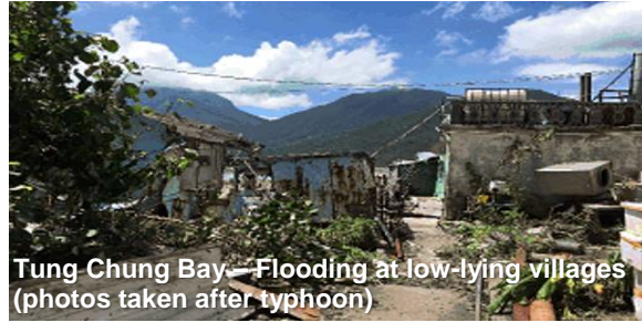
Tung Chung Bay – Flooding at low-lying villages (photos taken after typhoon)
