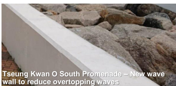
Tseung Kwan O Waterfront Park – New wave wall and pavement upgrades
