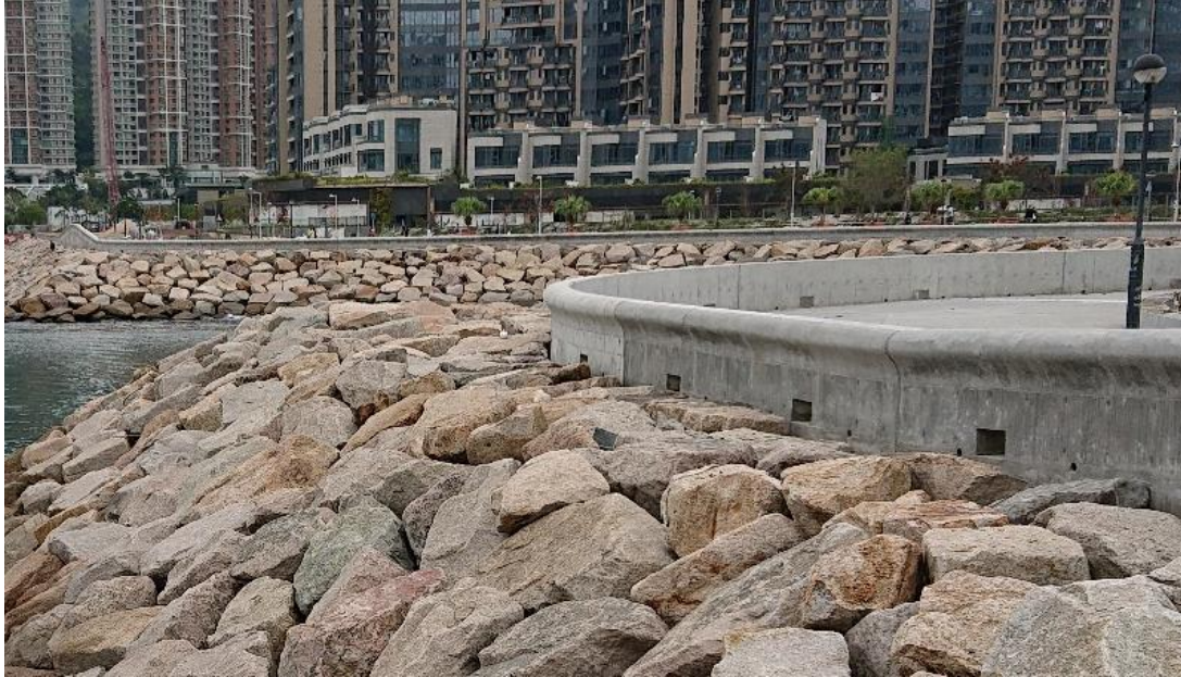
Plate 3-1: Rubble mound sloping seawall
