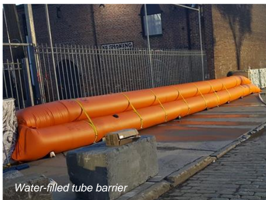
Demountable flood barrier around building
